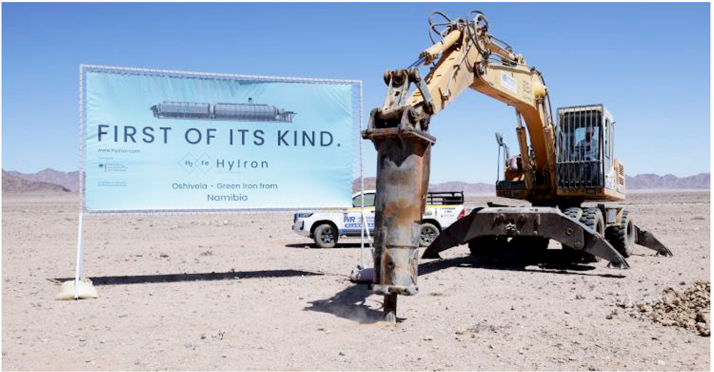
Photo: Hylron groundbreaking from Namibia Investment Promotion & Development Board
