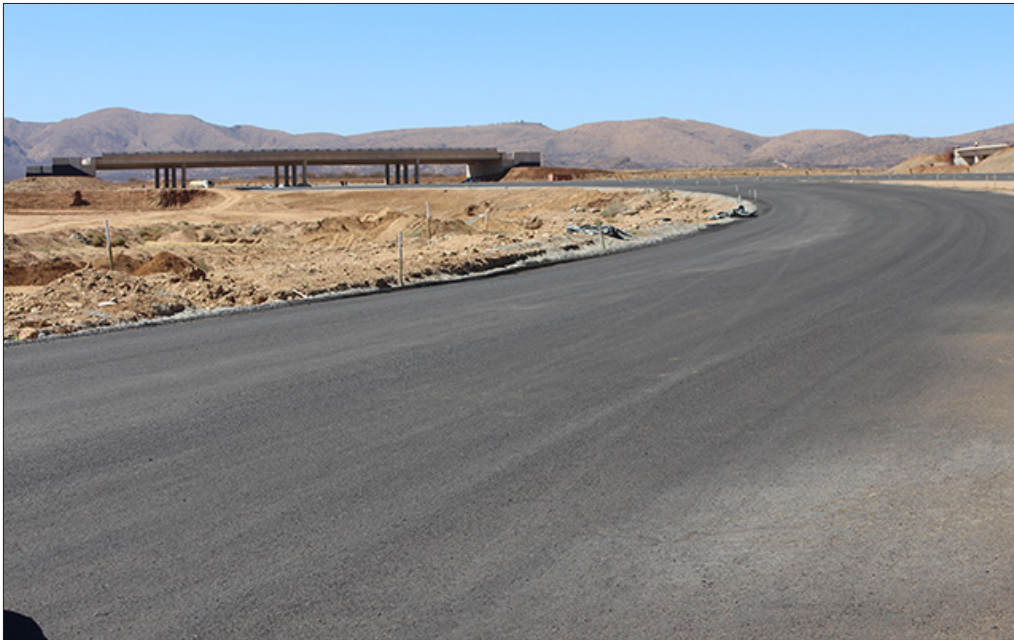
Part of the first phase road works of the Windhoek-Hosea Kutako International Airport dual carriageway.
