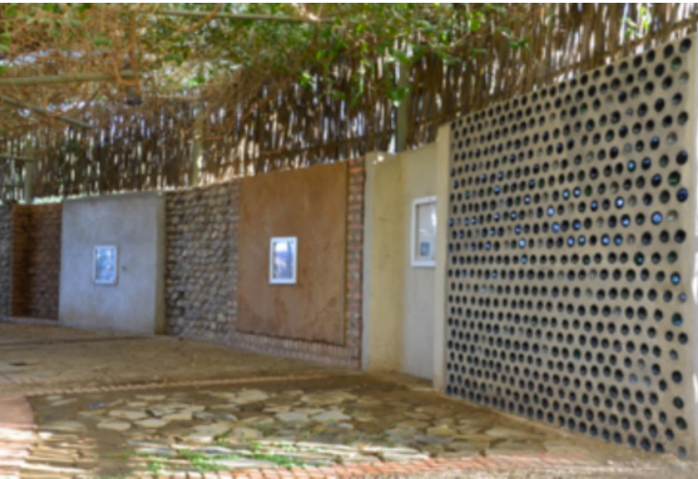
Different materials used for constructing walls at the HRDC
